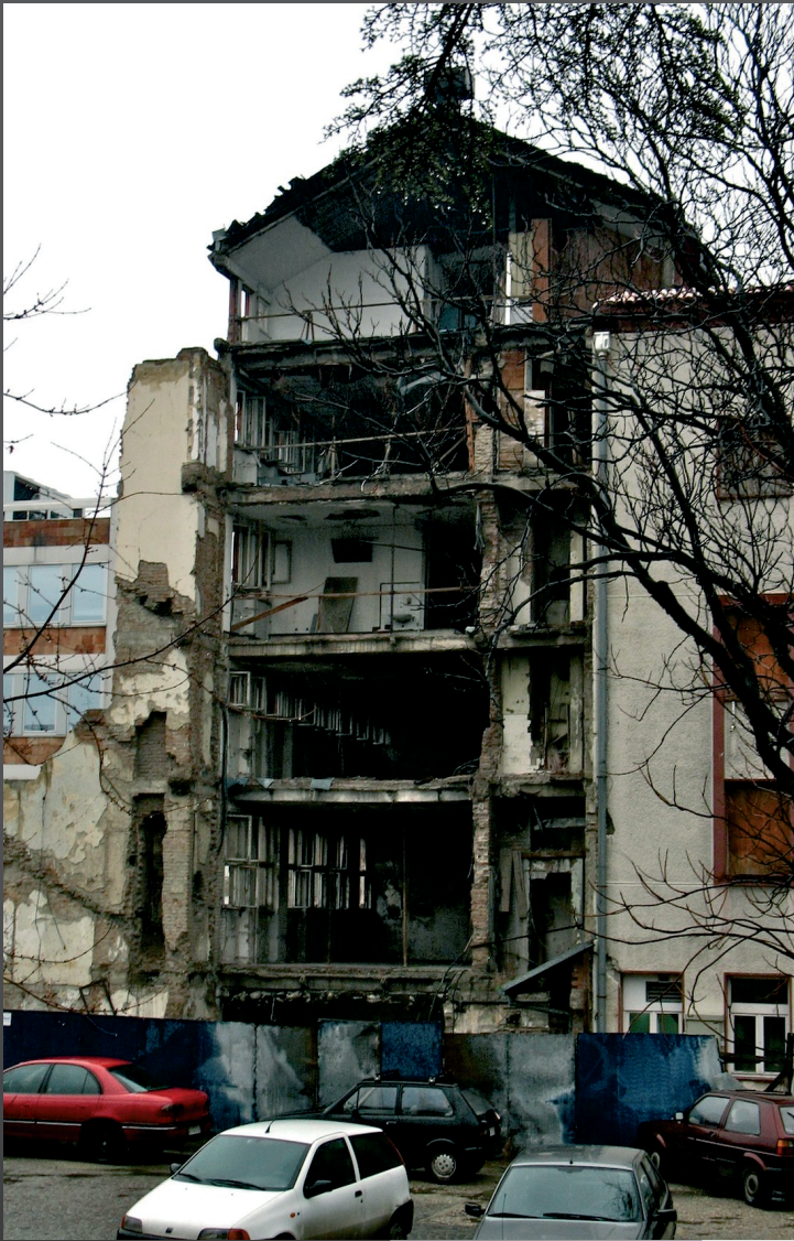
The building of the Radio Television of Serbia destroyed by NATO strike on April 23, 1999
