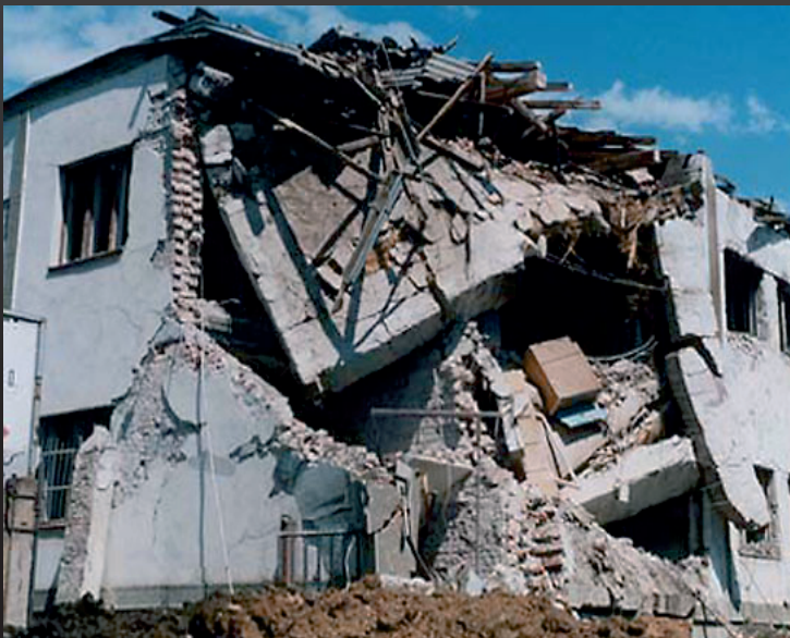
Destructions in the city of Niš resulting from the NATO airstrikes in 1999
